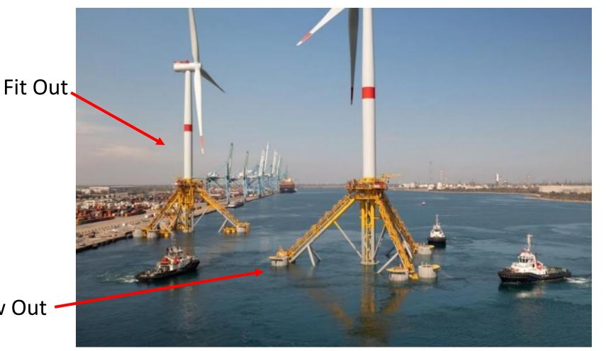
WTGs (and their associated substructures) will need to be temporarily stored in port until deployment becomes possible during an appropriate weather window, [2] and [3]
